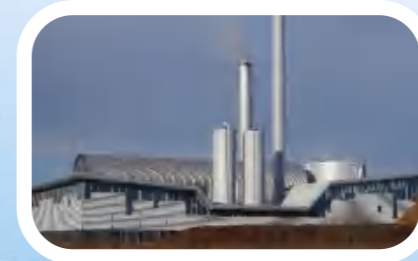
Sonderborg City Heating Station
