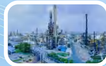
Jiujiang Coking Group.
